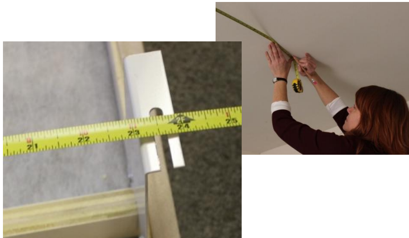
Measure & mark toggle bolt placement on ceiling 23.5" apart
